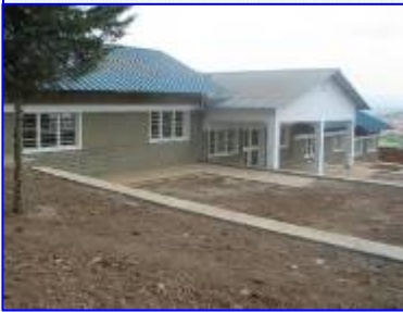
New constructed TBIF Incubator Buildings
